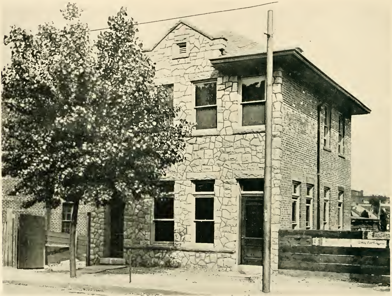
NEWARK PAVING CO., FIRST STREET
